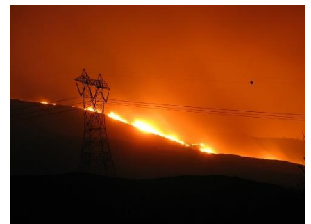
Wildfire near power lines
